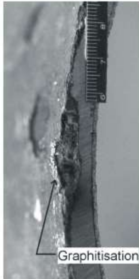
Figure 5. Cross-section of ductile iron pipe showing graphitisation. (City of Ottawa)
