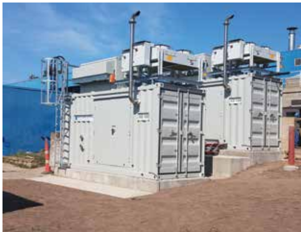
Twin KB 100 Biogas CHP Modules Pictured above
