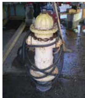
Figure 2: Four-connection manifold bulk water fill station off of a fire hydrant with no backflow protection.
